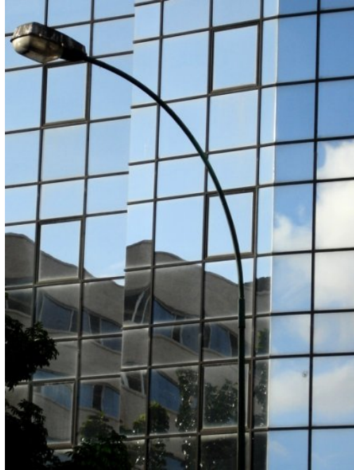
Figure 3. Distortion caused by glass outside the facade plane.
